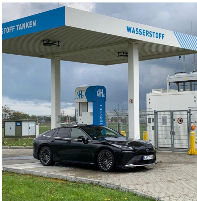
At this hydrogen station, the refrigeration machine with the hydrogen treatment is clearly visible in the background. (©: H2 Mobility)
