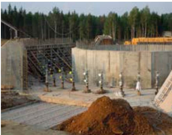
View of the construction site
